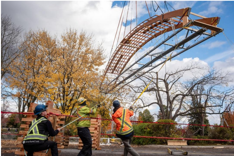
Confederation Drive Pedestrian Bridge
